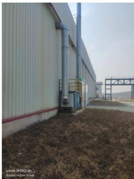
DA009 废油泥库排气筒
